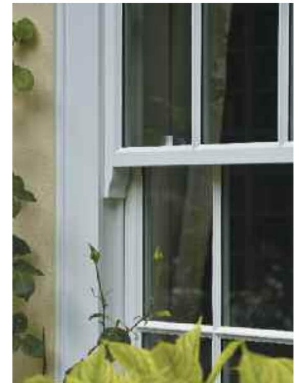
*Slim sash windows hung on traditional cords and weights mechanisms, finished in White with 14mm ultra slim, putty finished double-glazed units and 24mm true bars.*
