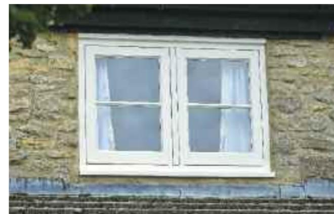
Replacing dark brown coloured windows, Mrs Grant opted for flush casement windows in a colour complementary to Farrow & Ball ‘Pointing’, a subtle, off-white shade. A simple horizontal 24mm true bar adds detail while 14mm ultra slim double-glazing units with traditional putty glazing, bring comfort and warmth.
