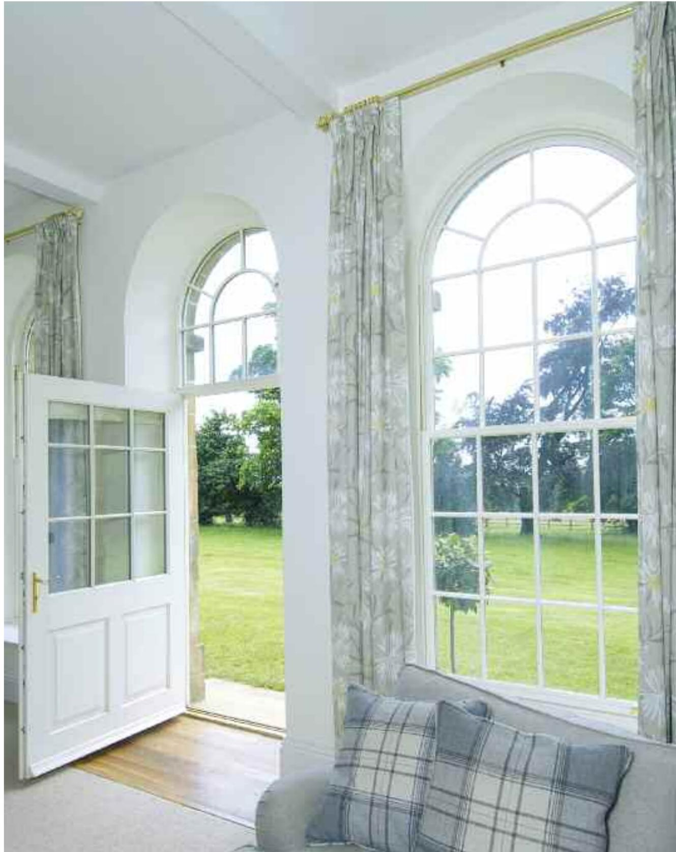
The new sash windows had to match the style and formation of the glazing bars from the original windows, the frames of which were still present once the openings were revealed.
