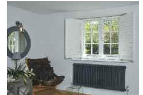
*Cottage flush casement windows, finished in 'White' with 4mm single putty glazing, 24mm true bars manufactured in Engineered European Redwood (14mm ultra slim double glazing to rear property windows)*
