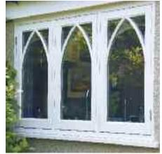
Of crucial importance to the acceptability of newly The 4mm single glazed pane and the ultra slim crafted windows and doors in historic settings, is the double glazed 14mm unit filled with krypton gas are hand finished with a traditional style putty and are available with a 22mm wide glazing bar, all features Referencing existing buildings and local style of
