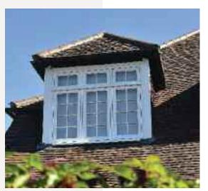
Flush casement windows finished in 'White' with 18mm astragal glazing bars and manufactured in Engineered European
