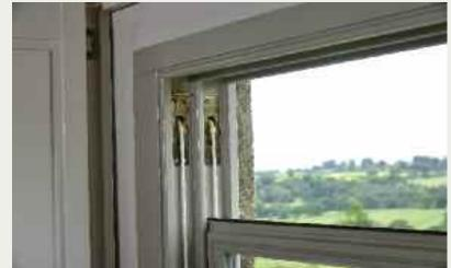
Slim sash windows with traditional cords & weights, finished in a colour complementary to Farrow & Ball 'Hardwick White' with 36mm astragal glazing bars and Mottled Antique Brass hook asteners and sash lifts.
