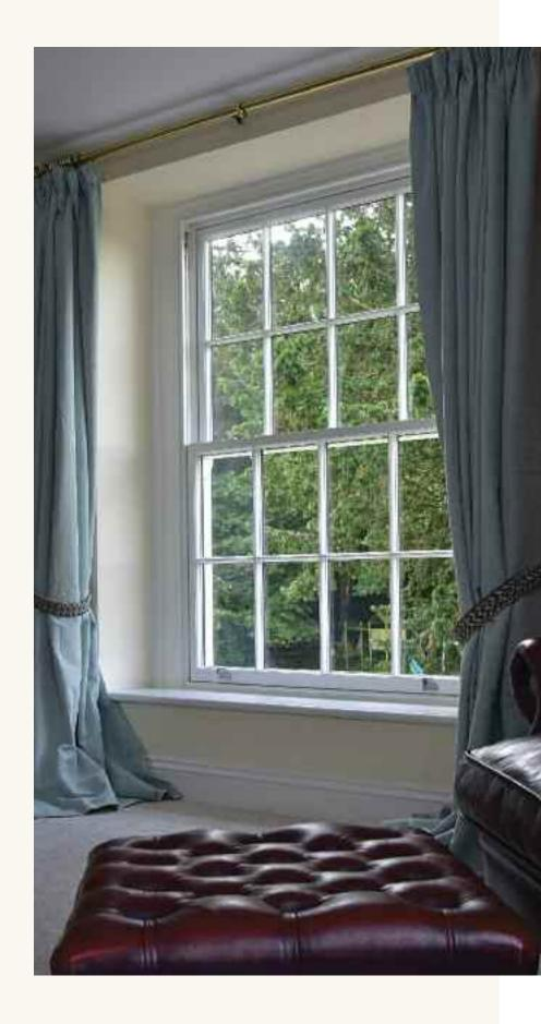
With the agreement that only the slimmest double glazing possible, would be permissible, the planning officer agreed to the solution on offer from Timber Windows; this being our 14mm ultra slim, krypton gas filled glazing units used for the various casement and sash windows throughout this impressive property.
