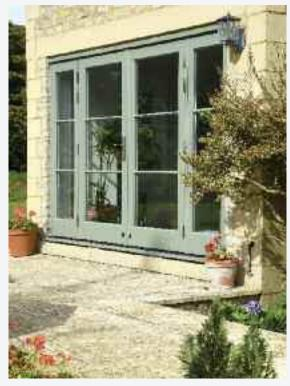
French doors with sidelights finished externally in Tent Grey' featuring 18mm astragal glazing bars and Pewter Avon handle. Manufactured in Engineered
